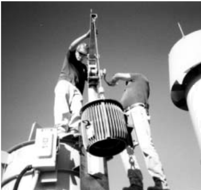
Lift new stator into place.
